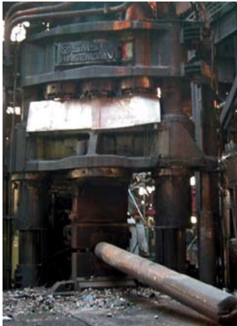
Condition of the open-die forging press after the fire
